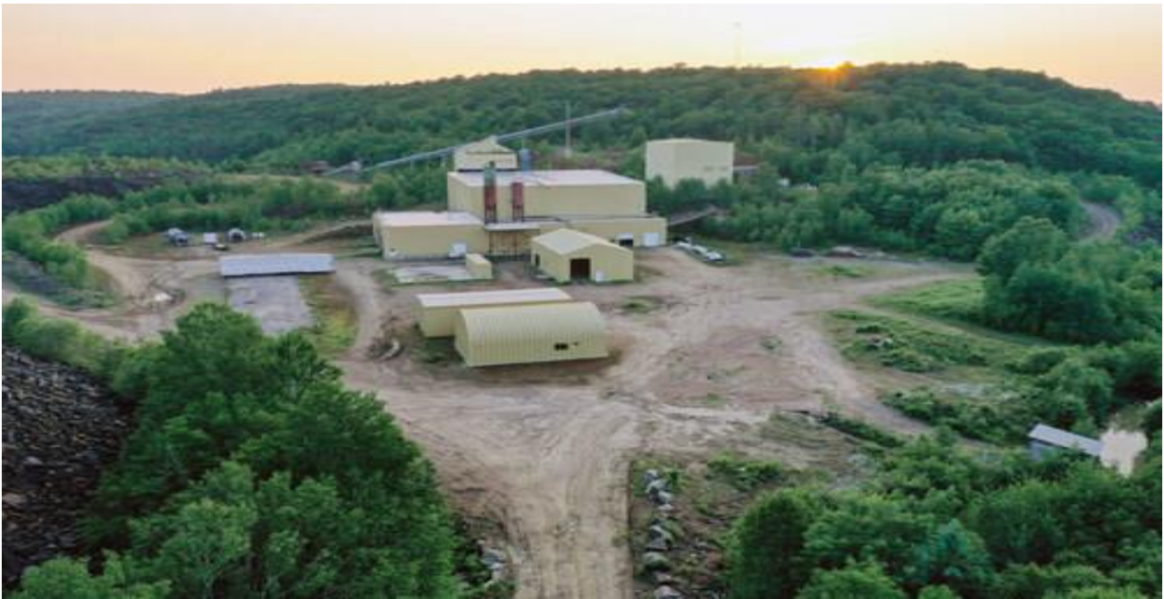
Figure 1 Mill Area Kearney Mine, Canada – Photo courtesy Global Battery Materials
