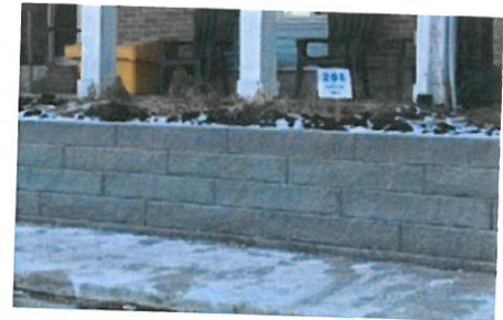
Retaining wall complete – Church Street
