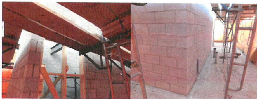
1 st floor West stairwell
