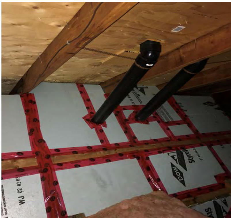
PHOTO OF ENCLOSED ATTIC FURANCE ABOVE GYMNASIUM
