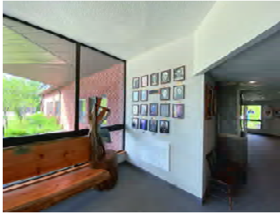
INT094 - Lobby Entrance Curtain Wall
