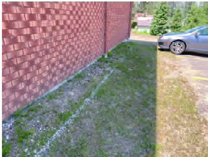
EX031 - Community Hall North Foundation Wall
