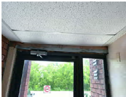
INT017 - Corridor East Exit Door Head
