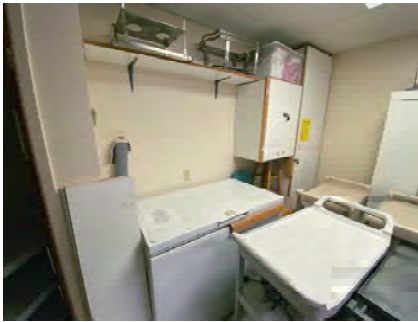
INT076 - Kitchen Storage Freezer
