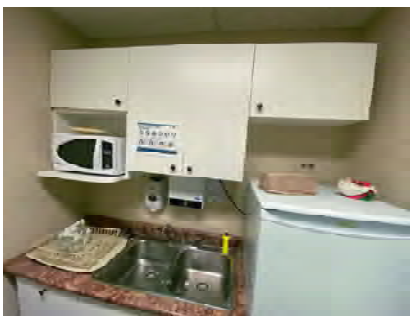
INT133 - Kitchenette Upper Cabinet Millwork
