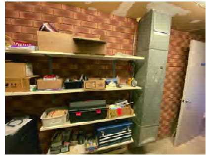
INT024 - Electrical Room looking South
