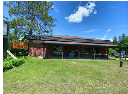
EX006 - Municipal Office South Overview
