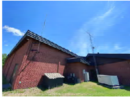
EX020 - Community Hall South Gymnasium Wall
