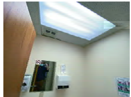
INT063 - Janitor Washroom Ceiling
