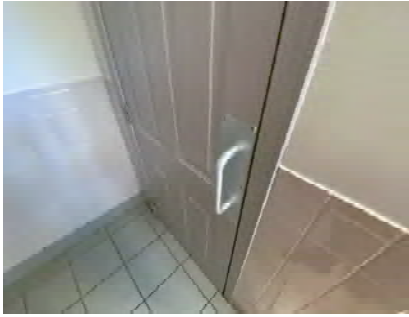
INT136 - Female Washroom Vestibule
