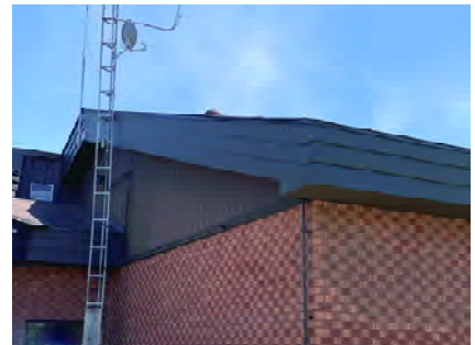
EX018 - Municipal Office North West Corner
