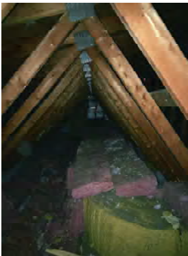
INT004 - Gymnasium Attic Space Insulated Ductwork
