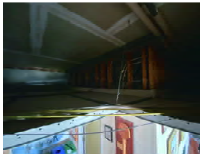
INT098 - Lobby Ceiling Space looking North
