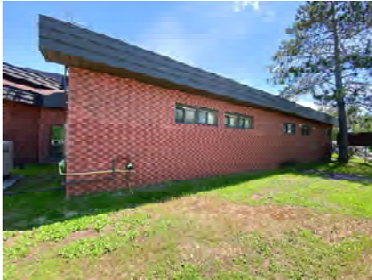
EX013 - Municipal Office West Exterior Wall
