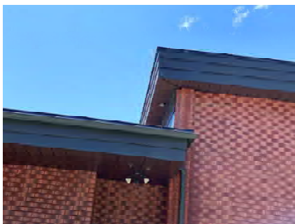
EX034 - Community Hall North Roof
