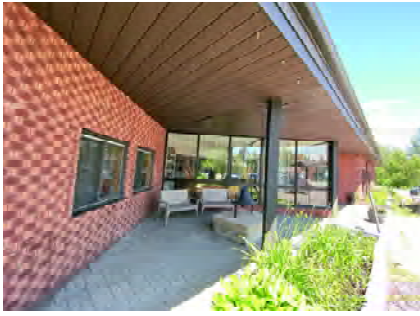
EX001 - Municipal Office East Overhang
