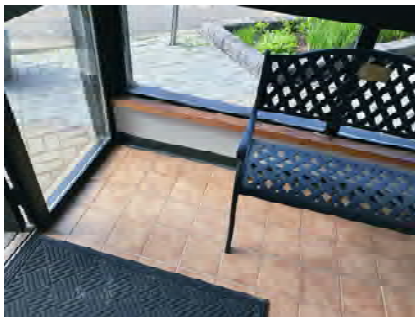
INT106 - Vestibule Floor
