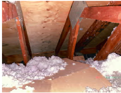
INT002 - Gymnasium Attic Space Roof Transition
