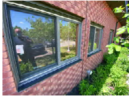
EX002 - Municipal Office East Exterior Wall
