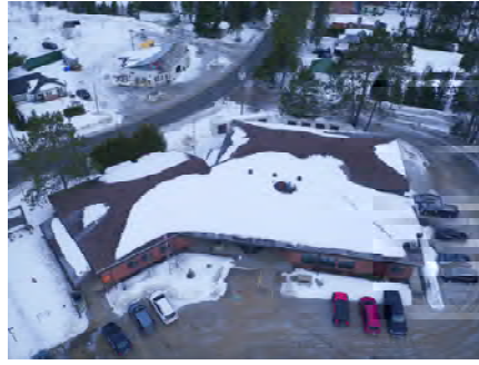
SITE029 - Aerial View looking West
