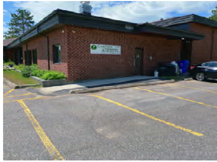
EX038 - Senior Club North East Exterior Wall
