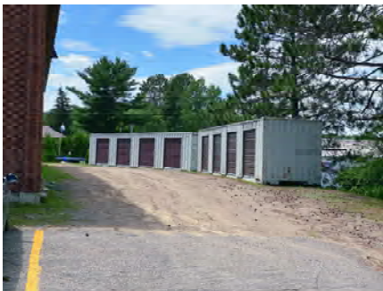
ES007 - Exterior Storage Container Overview
