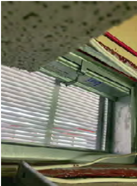
INT121 - Corridor Above Ceiling towards Library
