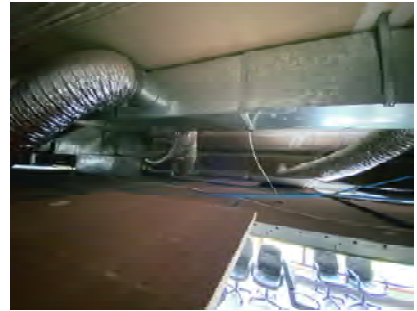
INT177 - Senior Lounge Ceiling Space
