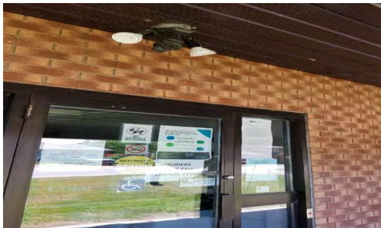
EXISTING EXTERIOR LIGHT FIXTURE WITH MOTION DETECTOR
