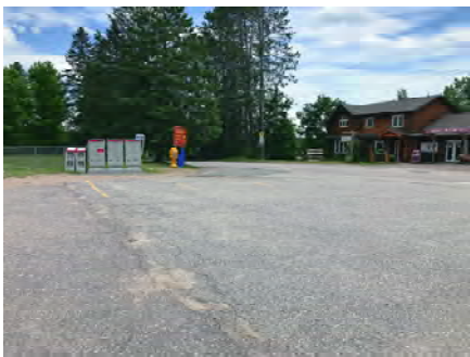
SITE004 - East Parking Area
