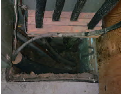
INT029 - Electrical Room Service Pit
