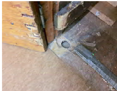
INT041 - Gymnasium Floor Construction
