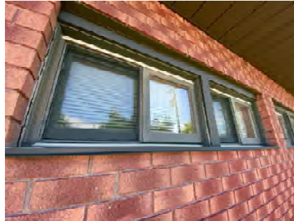
EX014 - Municipal Office Typical Washroom Window
