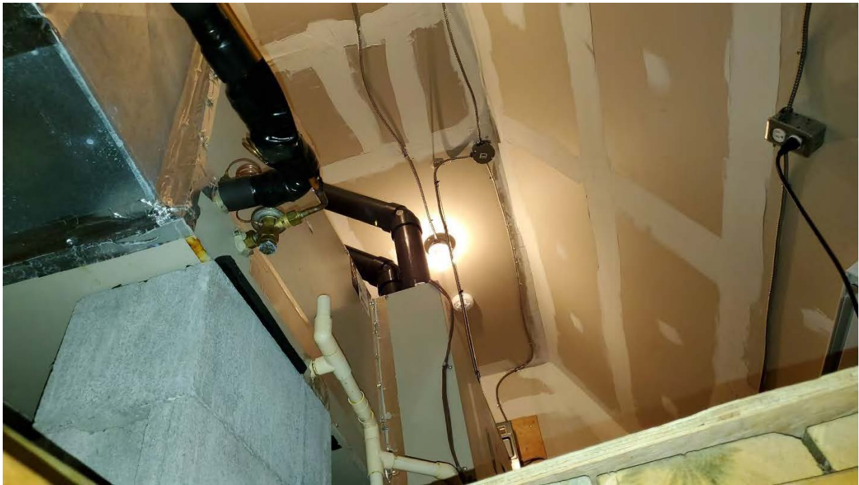
Figure 4: Municipal Office: Loft above the original flat roof framing.
