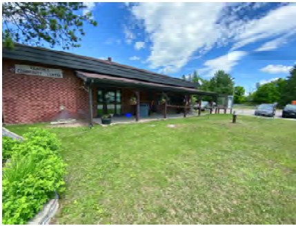
ES001 - Exterior Overhang Overview
