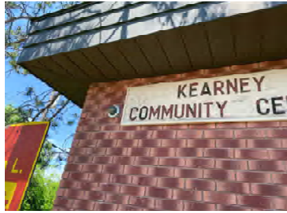
EX011 - Municipal Office South West Corner
