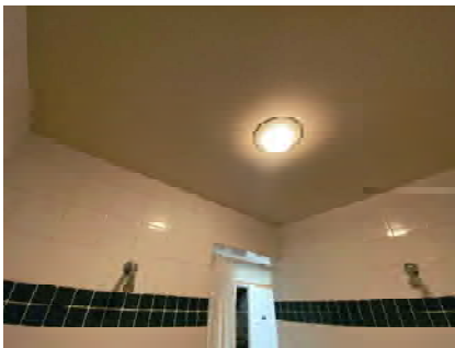
INT061 - Janitor Storage Shower Ceiling
