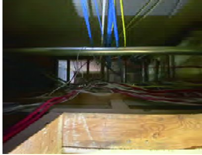
INT028 - Electrical Room Ceiling Plenum looking South
