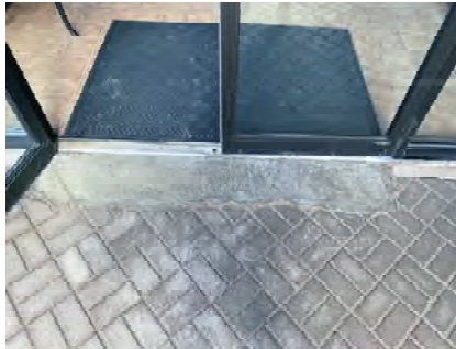
INT104 - Vestibule Main Entrance Door
