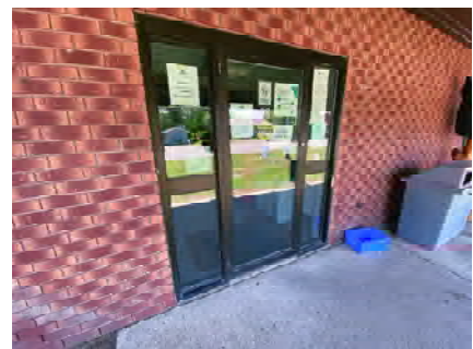
EX009 - Municipal Office South Exit Door
