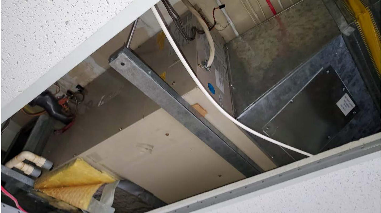
Figure 23: Community Hall Addition: Mechanical unit suspended from roof framing.
