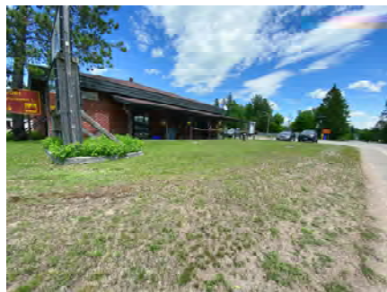
SITE008 - South West Site Area Looking North East
