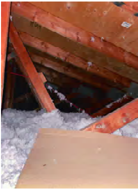
INT001 - Gymnasium Attic Space Trusses
