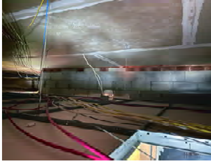
INT100 - Lobby Ceiling Space looking South
