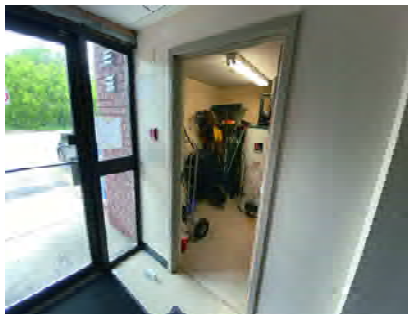
INT088 - Storage and Mechanical Room Door
