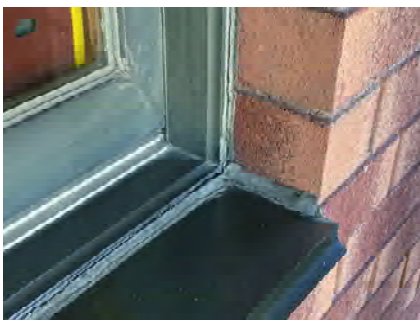
EX007 - Municipal Office South Service Window Sill
