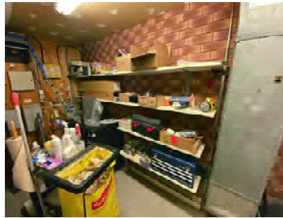
INT023 - Electrical Room Overview looking East
