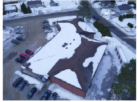
SITE030 - Aerial View looking South
