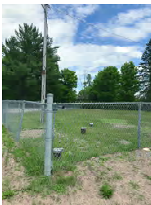
SITE007 - Septic Field Bed
