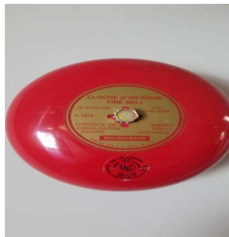
EXISTING FIRE ALARM SIGNALING DEVICE
