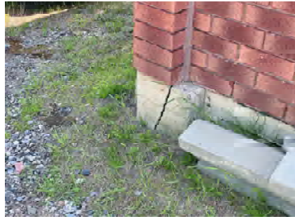
EX029 - Community Hall Gymnasium Foundation at North West Corner
