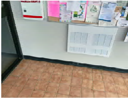
INT109 - Vestibule looking towards Senior's Club
