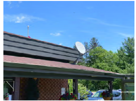
ES003 - Exterior Overhang Roof
