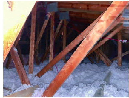
INT003 - Gymnasium Attic Space Typical Joist Insulation
