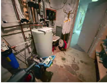
INT150 Mechanical Room towards Corridor Door
