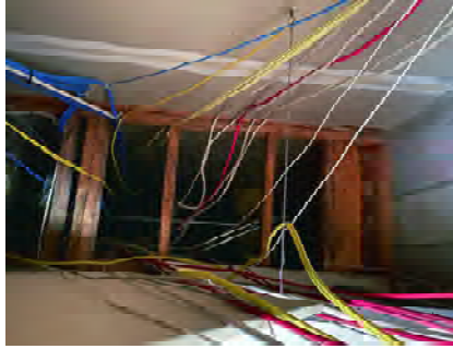
INT101 - Lobby Ceiling Space looking towards Electrical Room
