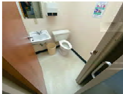
INT062 - Janitor Washroom
