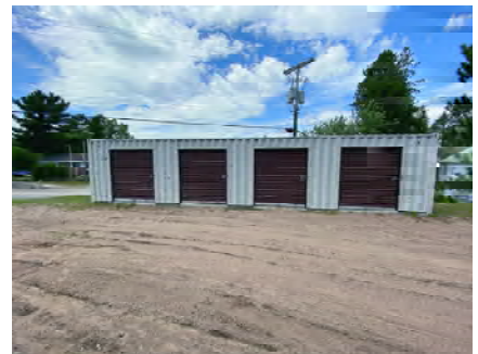
ES009 - South Exterior Storage Container
