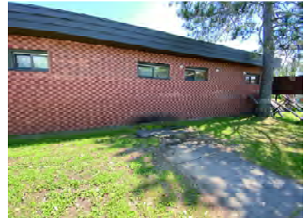
EX012 - Municipal Office West Exterior Wall
