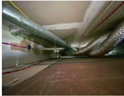
INT176 - Senior Lounge Ceiling Space
