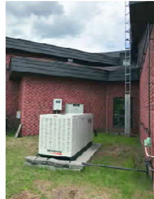
SITE015 - West Site Area looking East
