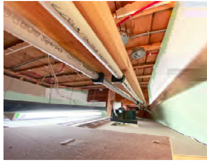
INT119 - Typical Ceiling Space Above Corridor
