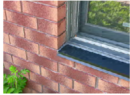
EX003 - Municipal Office Typical East Window Sill
