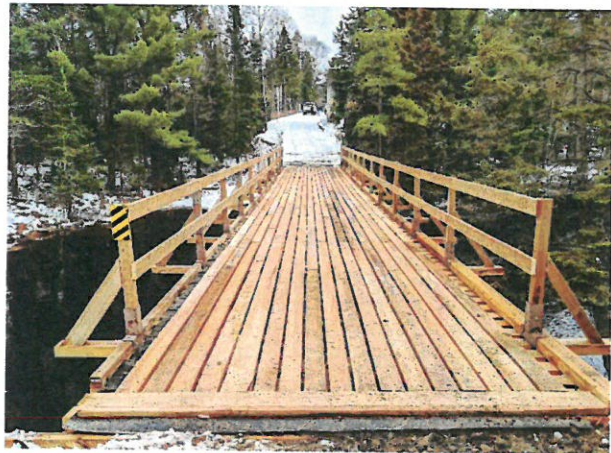
Seguin Falls Bridge completed Nov. 20, 2019
