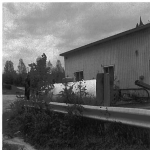
Photograph 7: Propane tank set back from building
