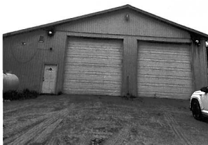
Photograph 1: Northwest (back) building elevation
