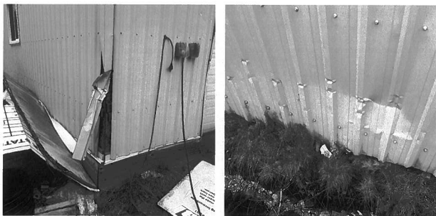
Photograph 23: Exterior siding impact siding
