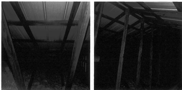
Photograph 11: General view of trusses in original building
