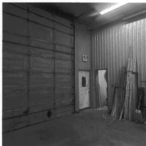
Photograph 16: Retrofitted/insulated section doors in west addition
