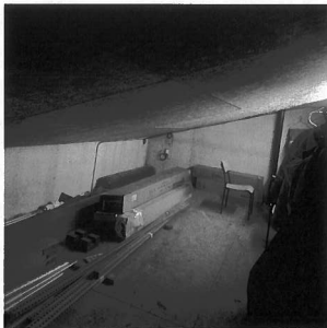
Photograph 15: Storage loft above office space, staffroom and mechanical room
