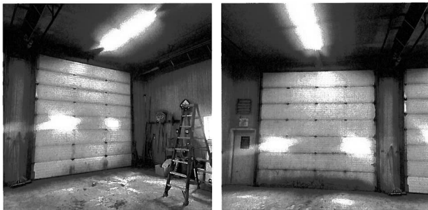
Photograph 9: Overhead doors of original building
