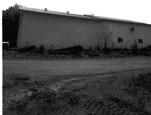
Photograph 2: Southwest building elevation
