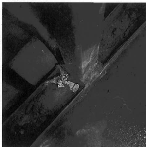
Photograph 20: Water accumulation and HSS column base corrosion
