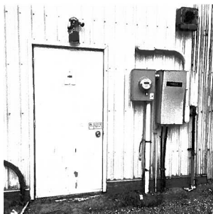
Photograph 14: Mechanical room access door
