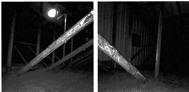
Photograph 17: General view of trusses in west addition
