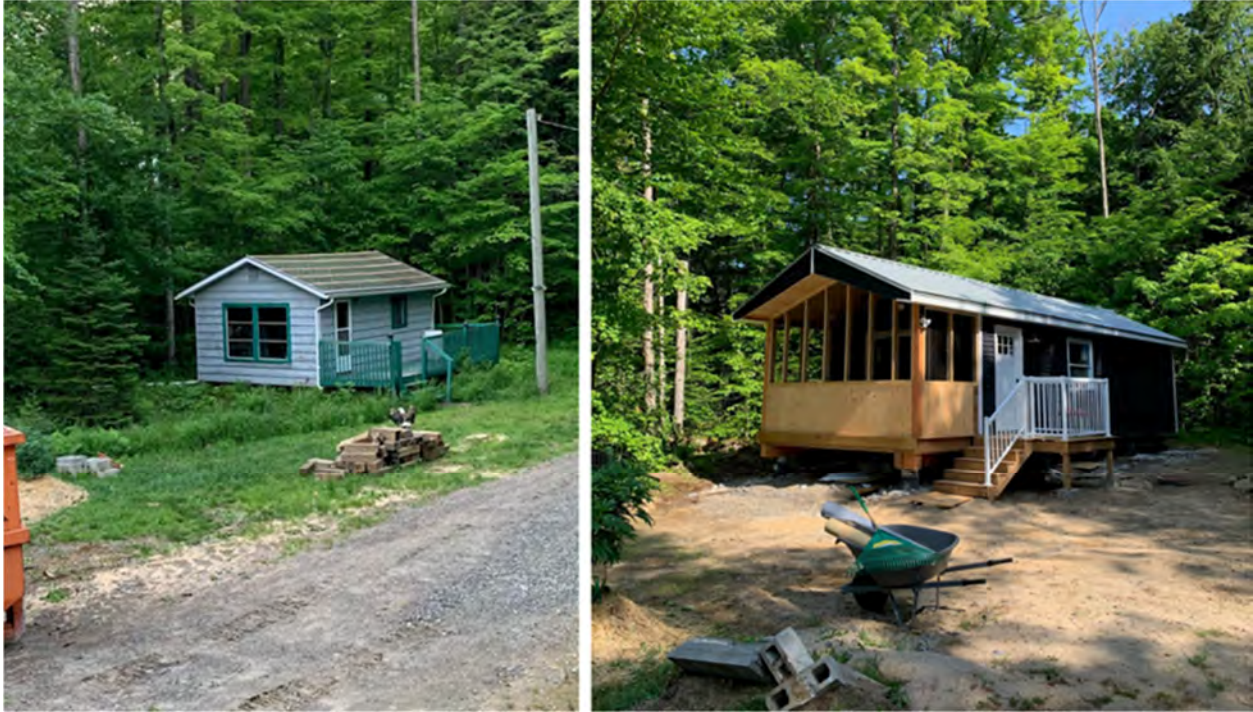
Figure 3: Old bunkie (left) and newly constructed bunkie (right).
